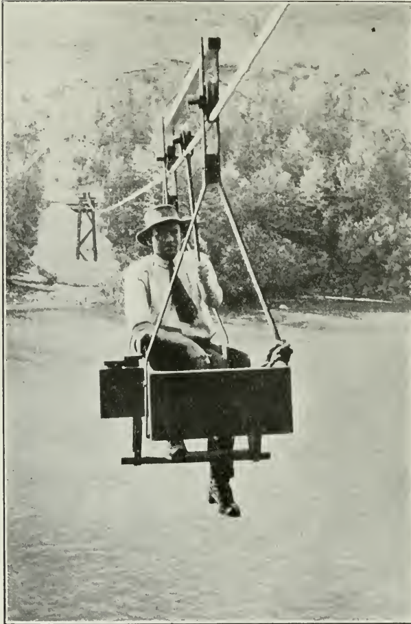
Cranbrook District (III).—Photograph showing cable car and method of operating.
