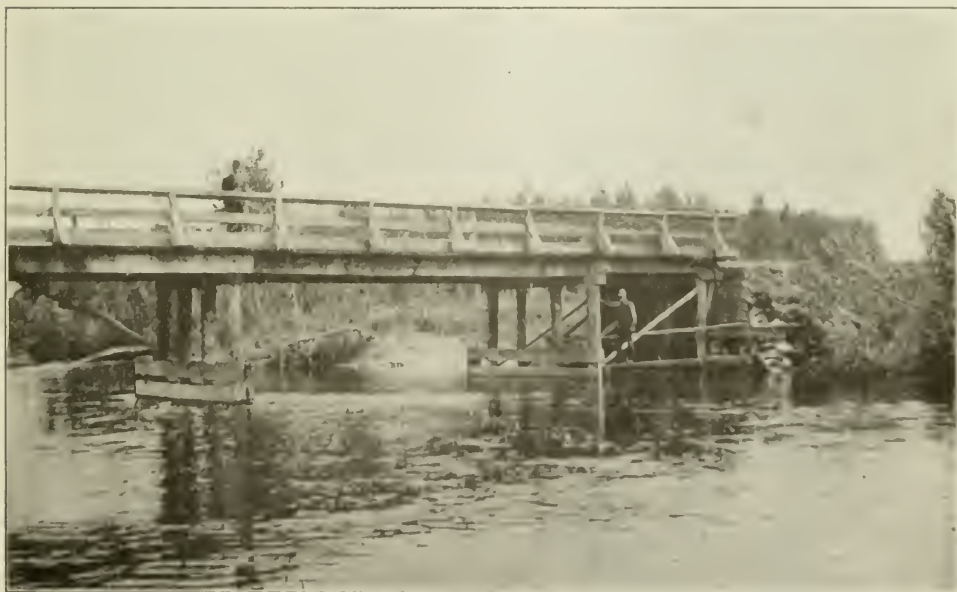
Brokenhead River, Sinnot. Bridge, showing gauge.
