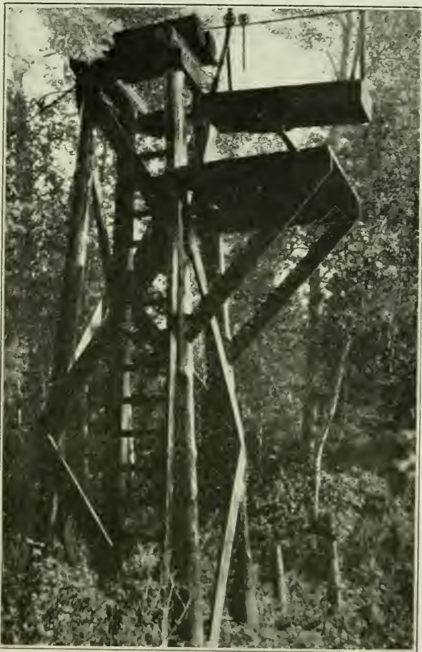
Cranbrook District (II)—Photograph showing support for cable way and platform attachment for cable car.
