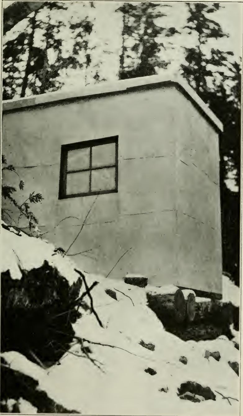
Adams River—Automatic Gauge House.
