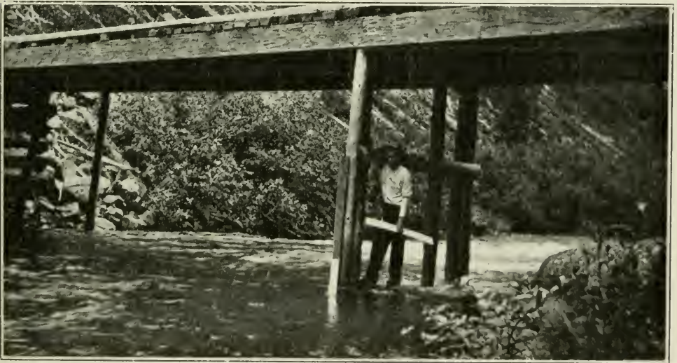
Installing metal-faced gauge at metering section on Sumallo river one mile from mouth.
