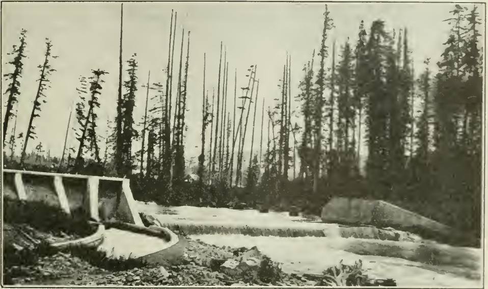
Diversion dam showing flume to intake, of Puntledge River Hydro-Electric Installation on Puntledge river about two miles below impounding dam.
