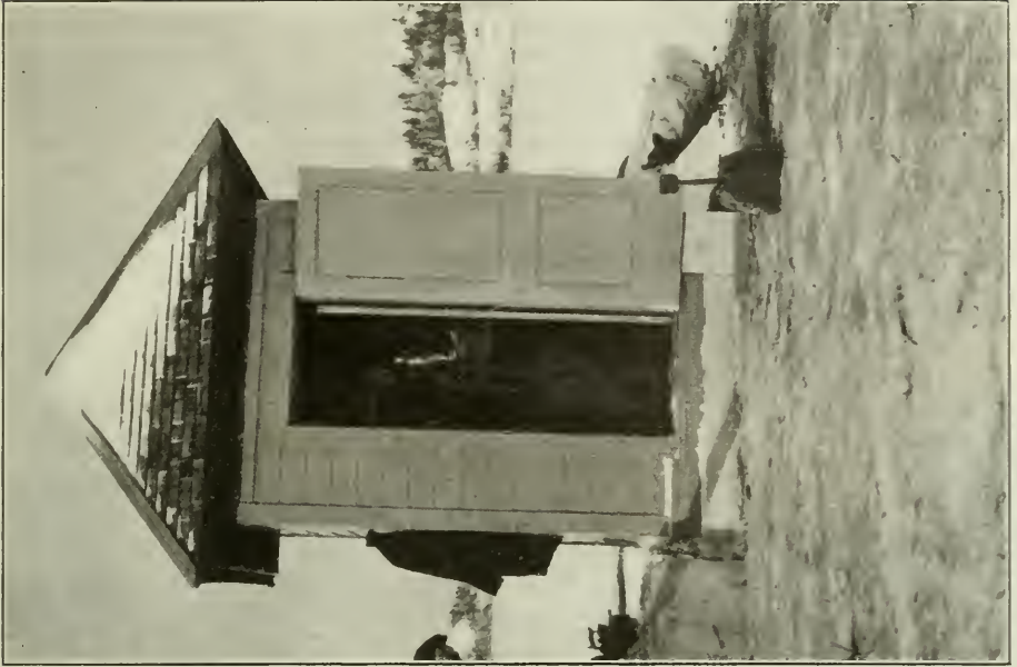
Automatic Gauge House, Kenora. Interior view.
