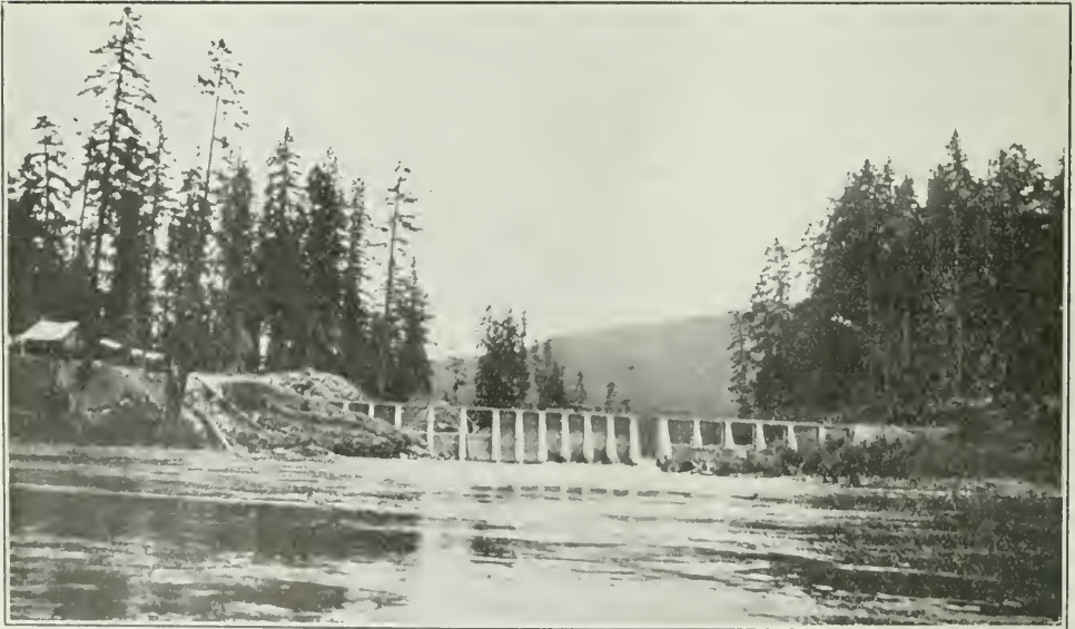
Impounding dam of Puntledge River Hydro-Electric Installation on Puntledge river near outlet from Comox lake.
