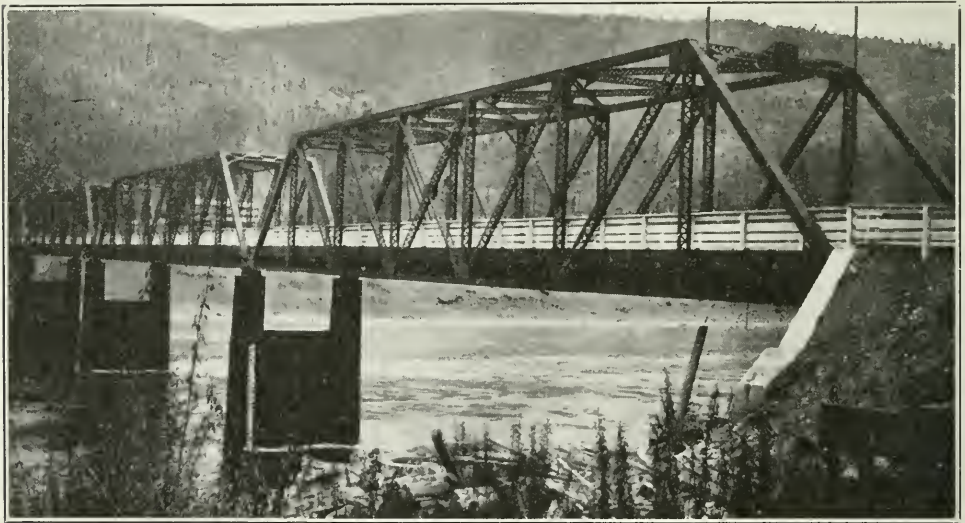
Nelson District (I)—Highway Bridge on Columbia river near Trail, showing metering section on upstream side of bridge.
