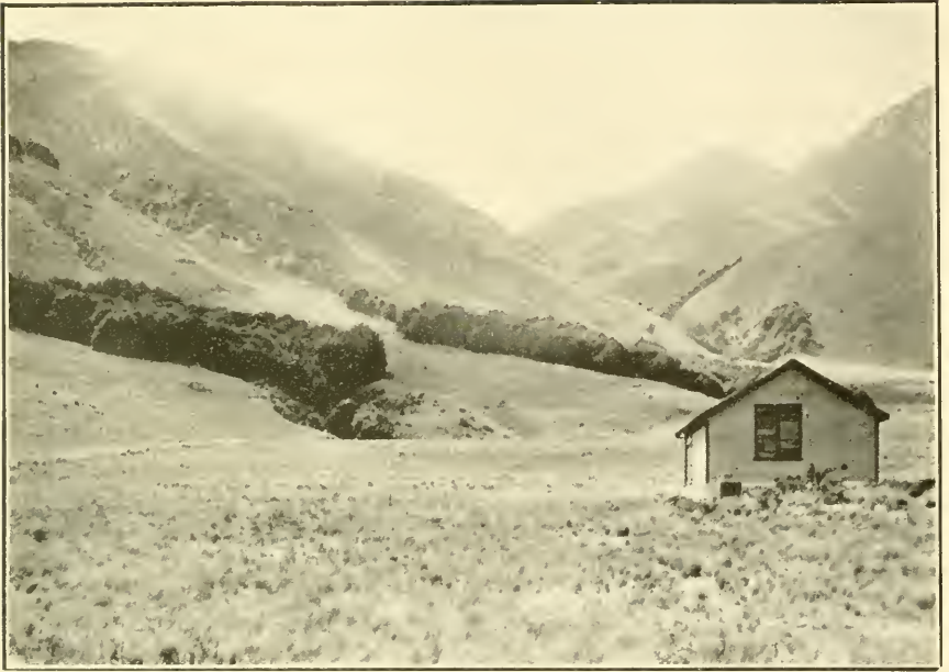
FIG. 3.—Station Building seen from the South-west.
