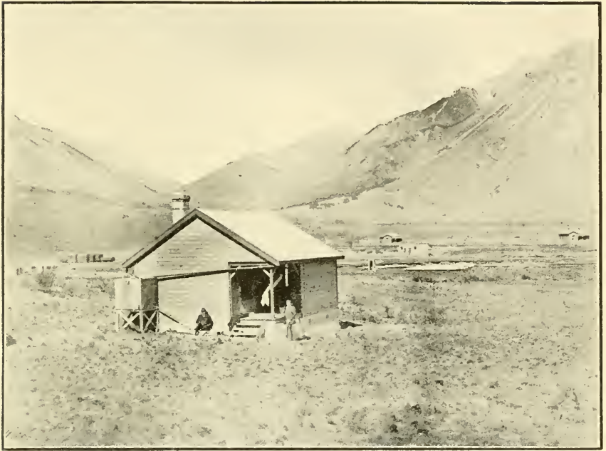
FIG. 1.—Station Building seen from the North-east.
